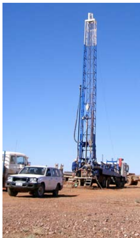
Drilling Welbourn Hill precollars - February 2008.
